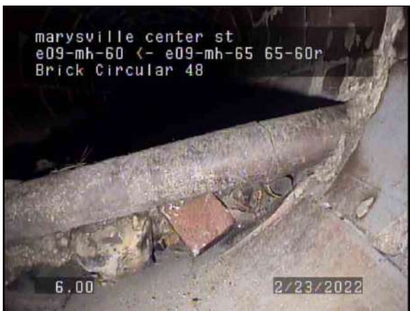
5, 00:04:12, 6.00ft Miscellaneous Survey Abandoned / reversal another cross bore
