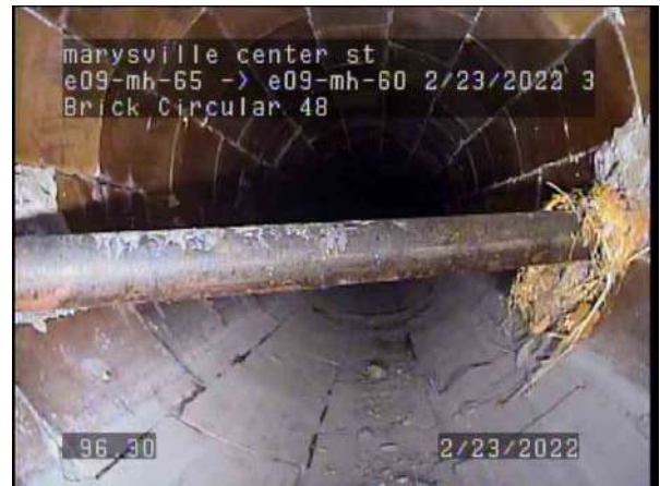
10, 00:05:19, 96.30ft Miscellaneous Survey Abandoned / cross bore
