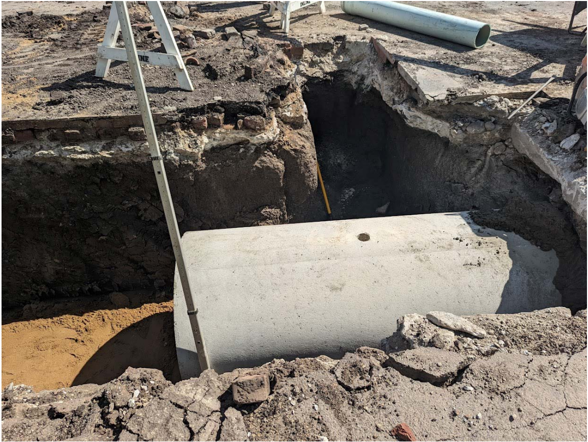
First section of new pipe installed
