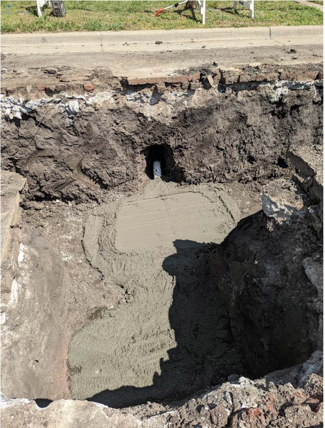
Sanitary service line covered in concrete.
