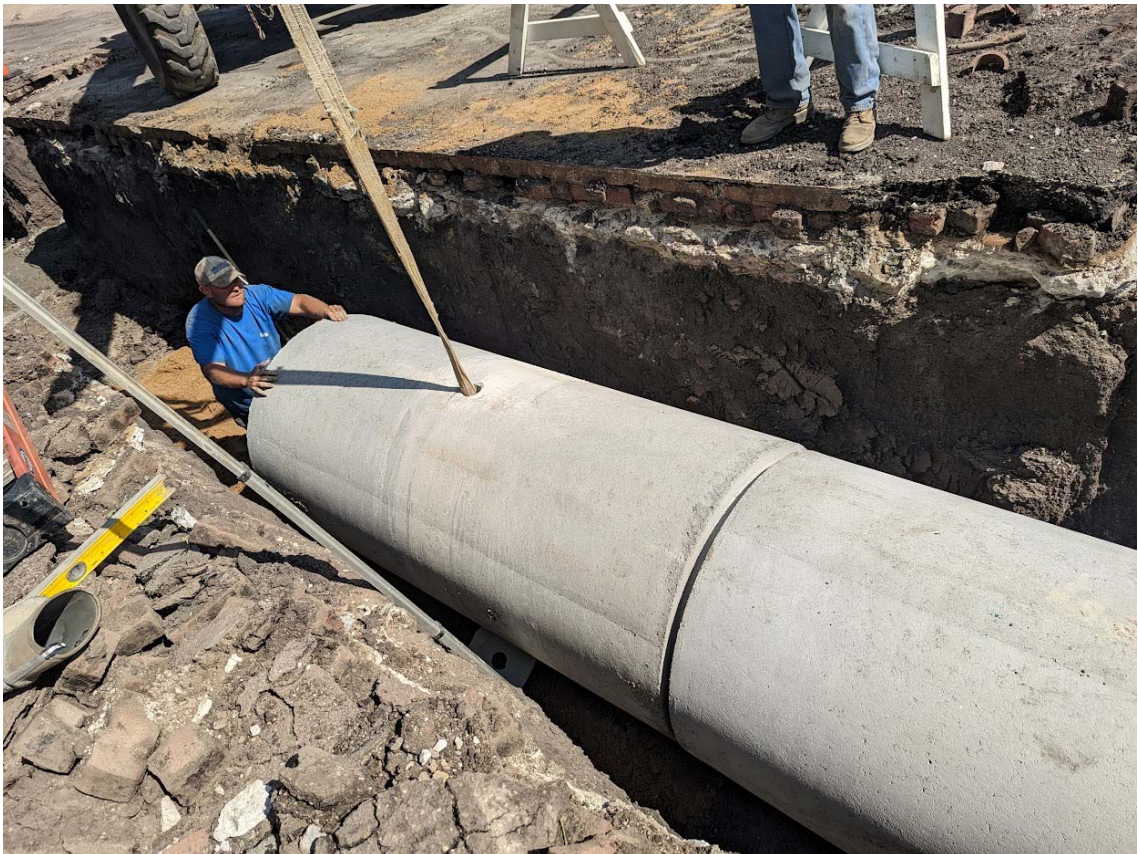
Second section of new storm sewer installed.
