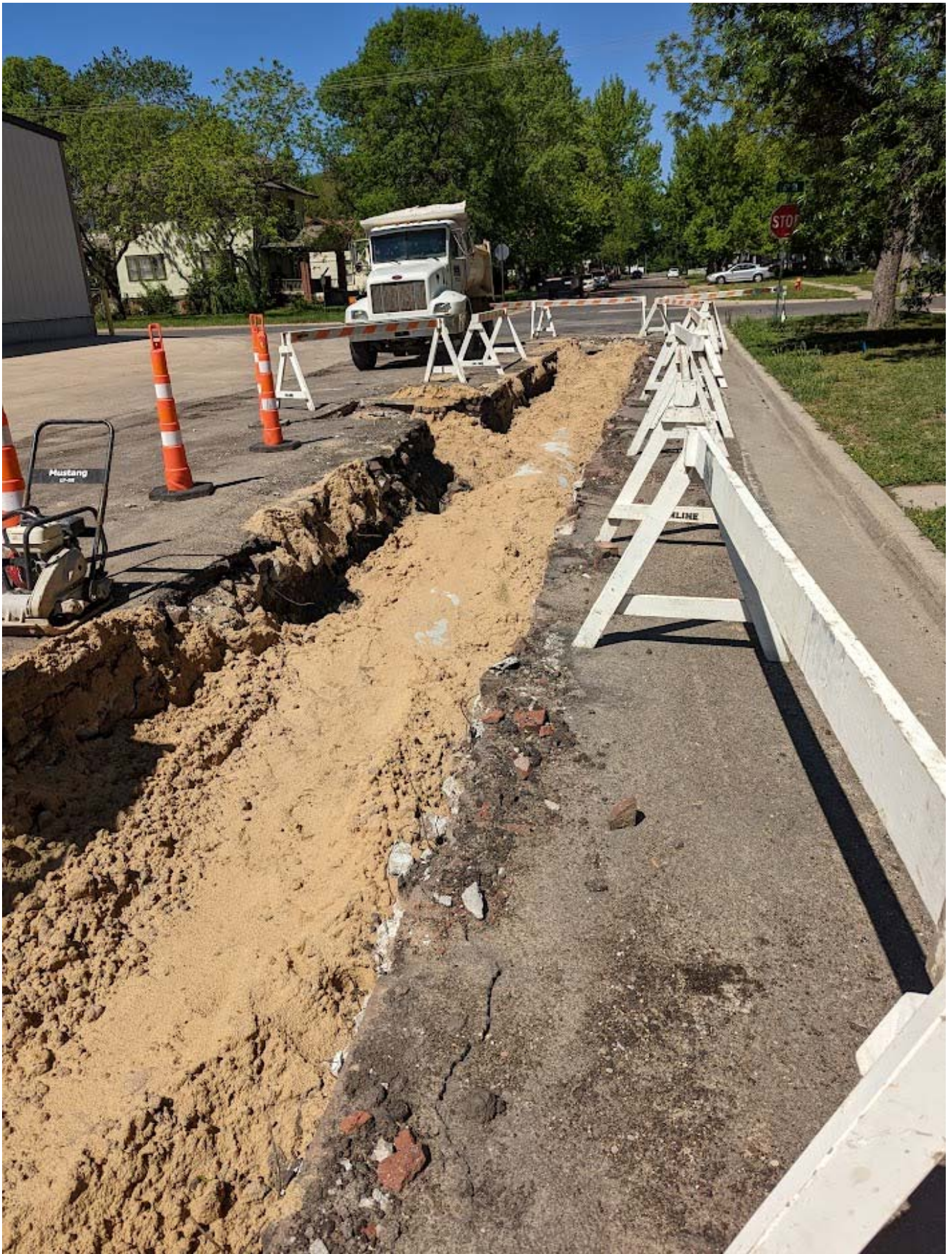
New pipe under sand.
