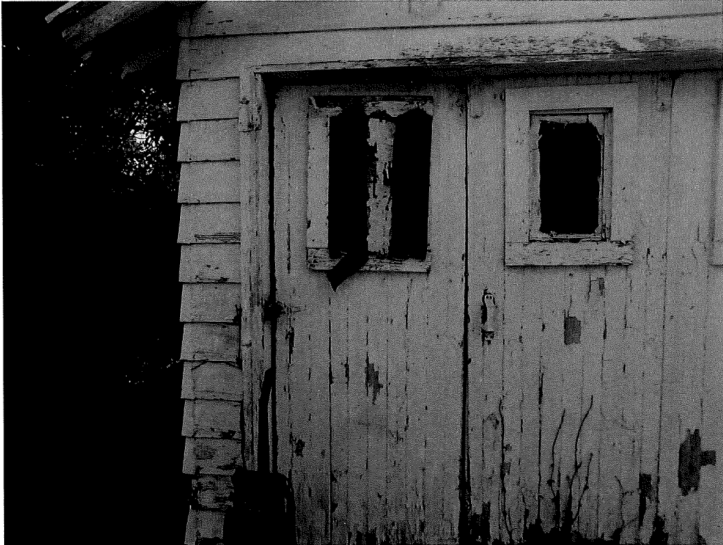
Top: Sheeting missing on west side Bottom: Window busted out. Door just leaning in hole
