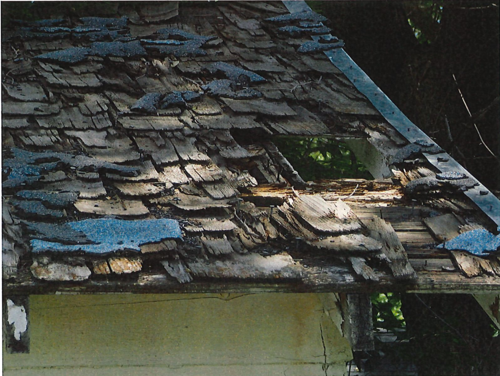
Top: Foundation on back wall is pushing out. Bottom: Hole in roof on east side
