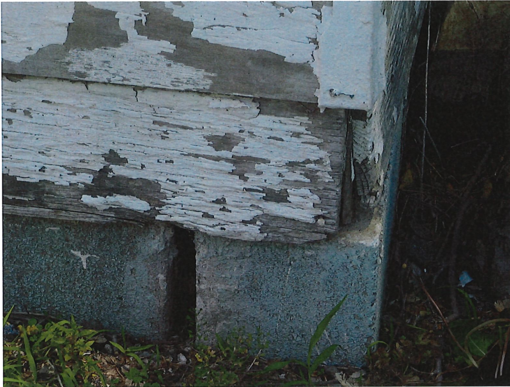
Top: Foundation on back wall is pushing out. Bottom: Hole in roof on east side
