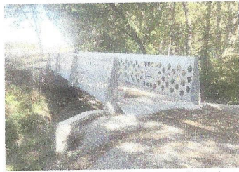
EXAMPLE: Existing Bridge at 7th & North Street
