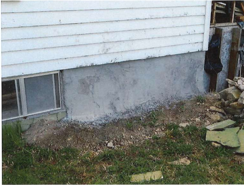
West side: Foundation of house repaired.
