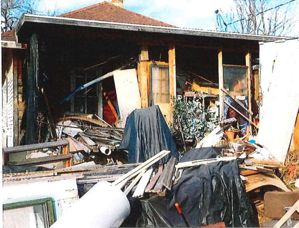
Miscellaneous Items Scattered across South porch and Yard
