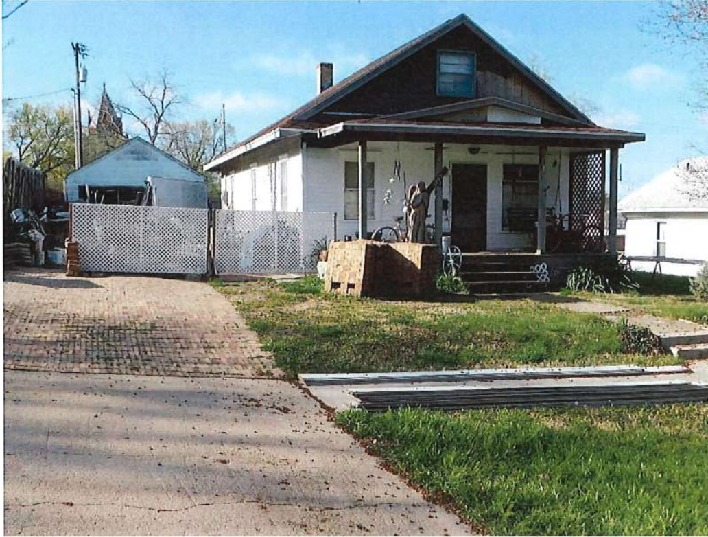
Top: front yard and porch cleaned up
